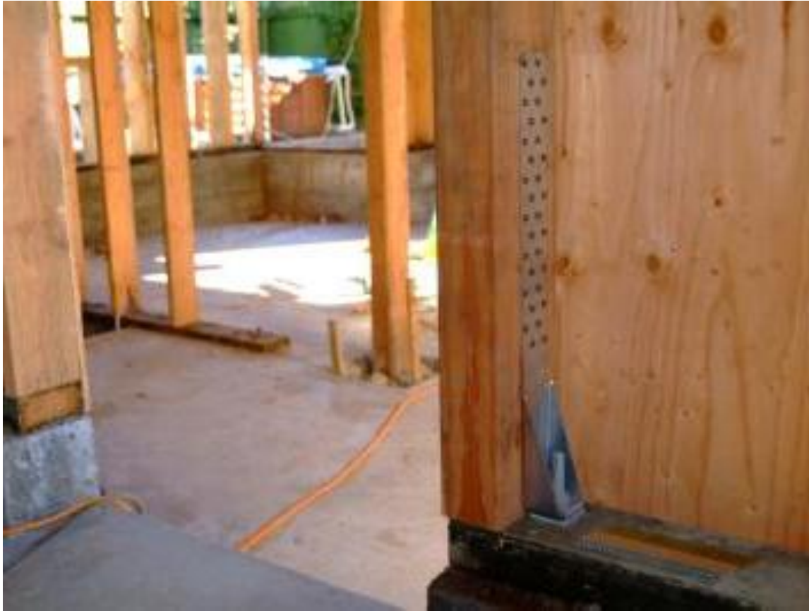
Napa CA, Feb. 14, 2006 -- Foundation bolts and straps are an inexpensive way to mitigate movement in the event of an earthquake. Photo by Adam DuBrowa.
