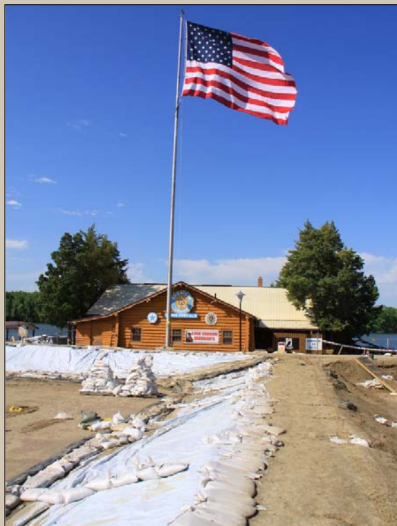
Preparing for rising waters in Pierre, SD (USACE / Harry Weddington)
